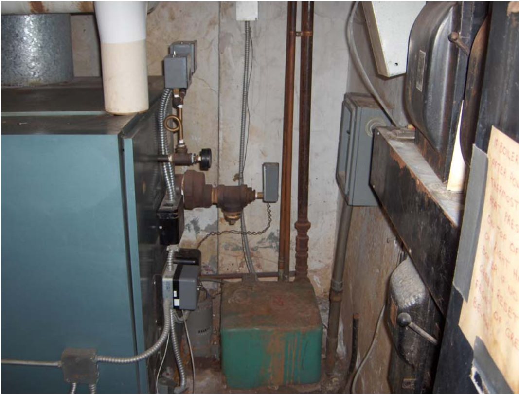
Right side of boiler – note re-set button in middle
