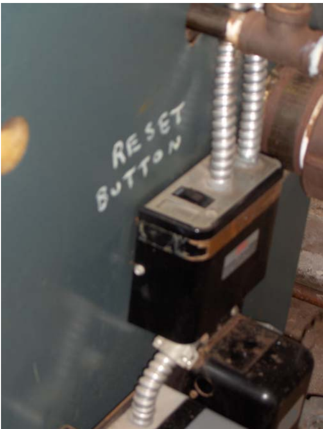
Right side of boiler – note re-set button in middle
